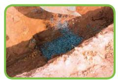
STEP 1: Excavate Drain Basin location to depth. Provide a stone base. (Width of excavation can be the same width as pipe trench)
