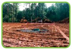
STEP 6: The drain basin body can be cut at the time of the final grade or raised with riser. No brick, stone or concrete block will be required to set the grate to the final grade height.
