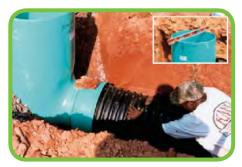
STEP 4: Backfill the back side of structures and push the pipe home to the seat position. Re-check Drain Basin depth, level and position.
