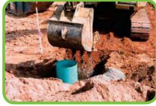
STEP 5: Backfill uniformly around structures with class I, II, or III material and compact in lifts according to ASTM D2321.
